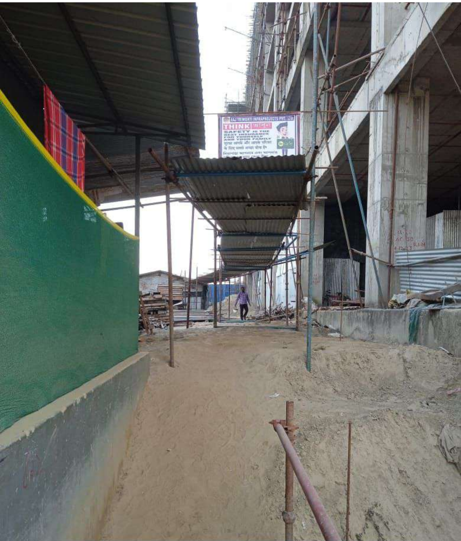
East wing building site zone
